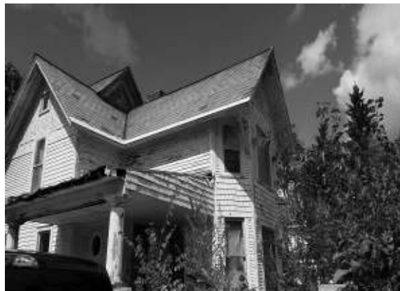
Photo #1: View of exterior of house (September 5, 2017)
