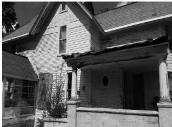
Photo #2: View of exterior of house (September 5, 2017)
